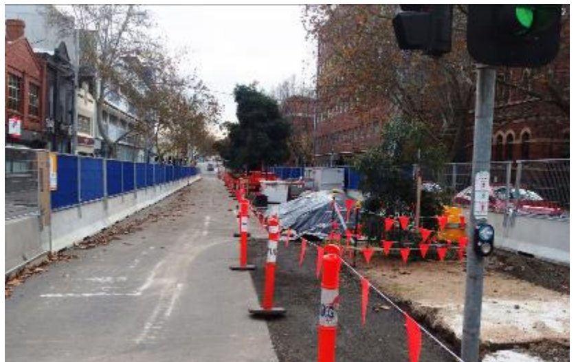
Queensberry Street make over in progress
