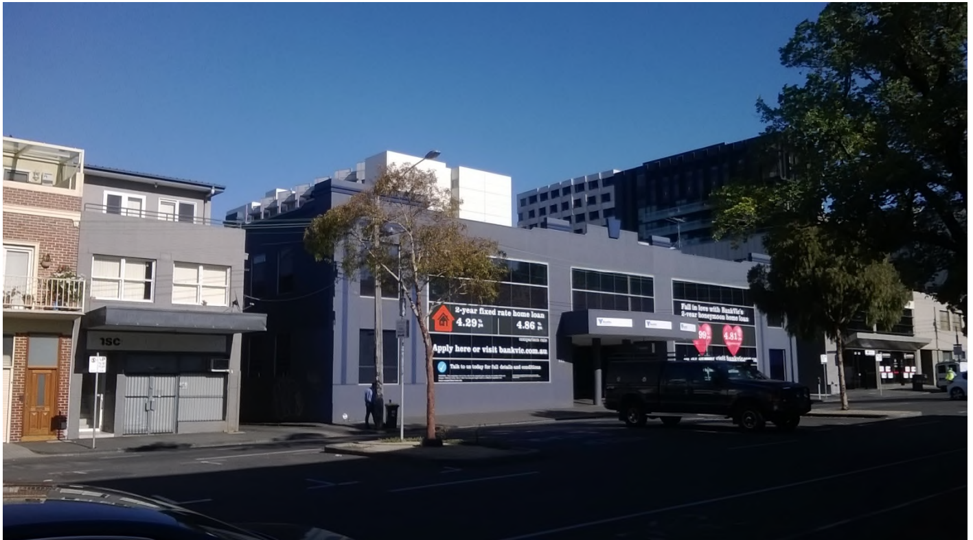
117 – 121 Cardigan Street, Carlton [to the rear of the subject site]
